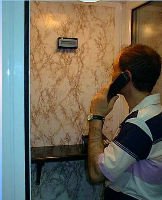
Fig.1.2. PLC module in post-office cabinet
